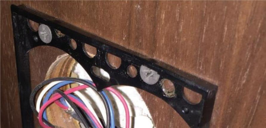
Photo 10: Example of improper screw used for surface mount installations.
